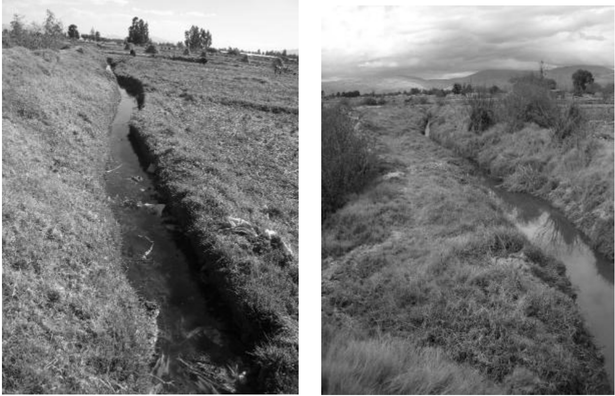
Figure 18. Open channels used to transport treated wastewater from the stabilization pond systems in Arani (left) and Punata (right) to the farms where it is used for irrigation.
